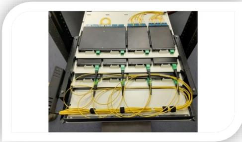
Rear – Loaded with MPO Trunk Cable. MPO's plug directly into cassettes.
